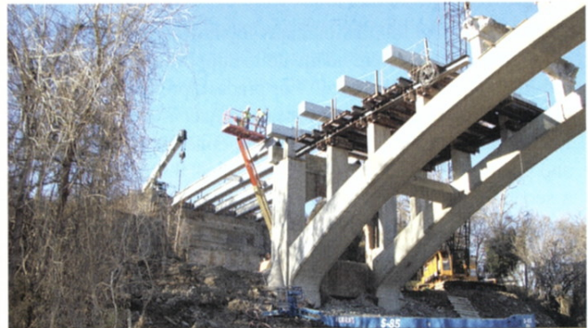
Precast spandrel beams were placed on top of the existing columns.
