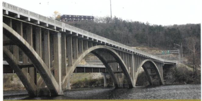
Photo of the completed bridge. All photos: Kevin Skibiski, Horner & Shifrin.
